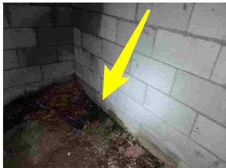
Water from cracked copper pipe
