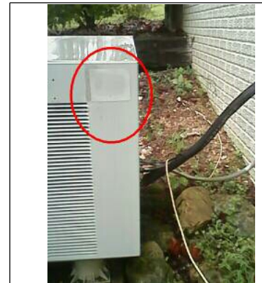
Faded \ missing label
