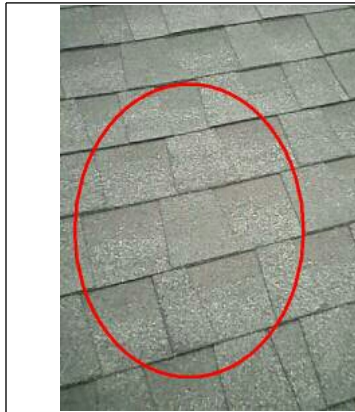
Missing granular
