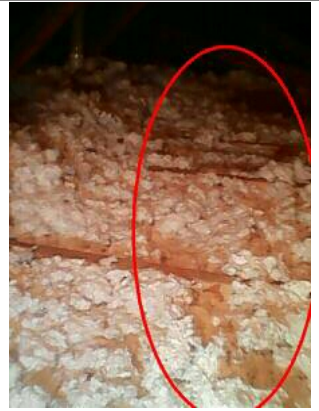
Compressed insulation
