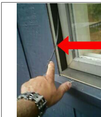
Kitchen window strip damage \ no screens
