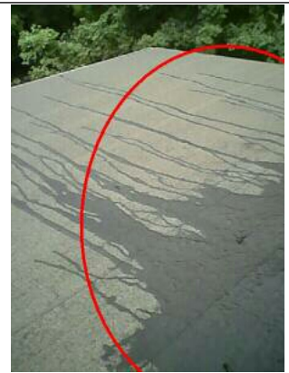
Tared over at chimney and rolled area west
