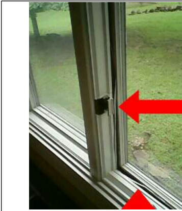
Weather stripping damaged
