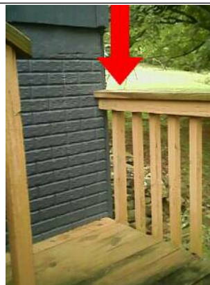
Loose, recommend bracing
