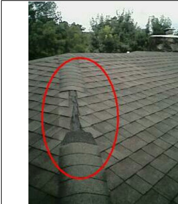
Carport Missing shingles on ridge
