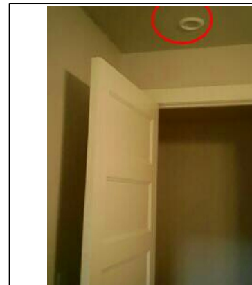
Missing smoke detector
