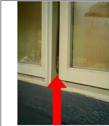
Loose weather stripping on several windows
