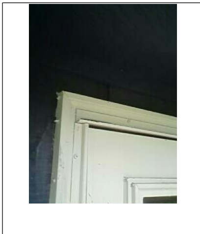
Drip edge flashing rusting, monitor
