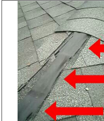
Missing shingles exposed felt
