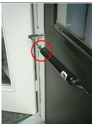
Tab does not hold screen door open
