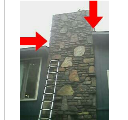
Recommend flashing to divert away from chimney
