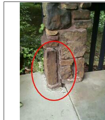
Loose stone, recommend repair
